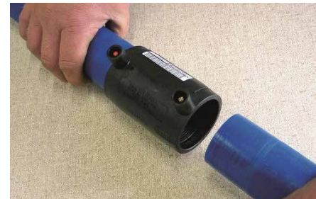
5. Assemble pipe and fitting making sure pipe is fully inserted, check witness mark. Clamps can be used to stabilise joint during welding.
