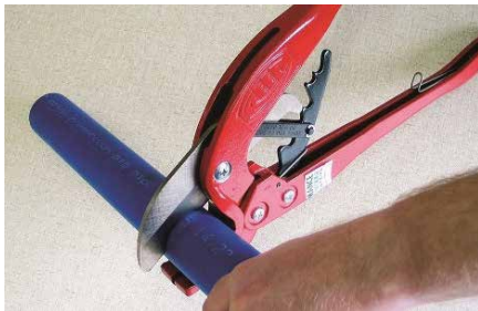
1. Cut pipe to length with approved cutters for a square swarf-free finish.
