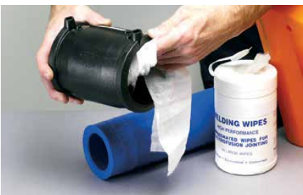
3. Use welding wipes to clean pipe and fitting surfaces. Allow cleaner to evaporate
