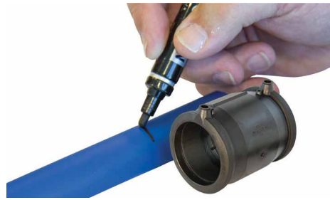
4. Witness mark correct insertion depth.
