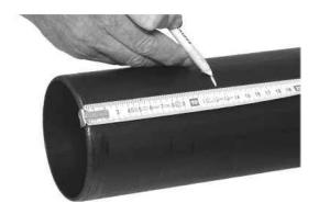
3. *Mark Insetion depth.*Use the insertion depth for the ambient temperature dusring installation
