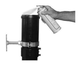
5. Install pipe and fix with a fixed-point bracket on the socket side and sliding brackets over the rest of the pipe length.
