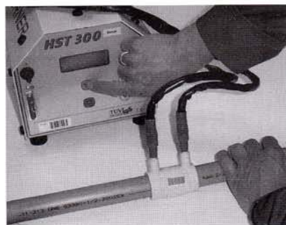
Fig. 7 Plug in the cable plugs in the contact bushings. Enter the voltage and the welding time in the welding device. The welding data can be seen on the barcode label of the socket. Start the welding device from the switch.
