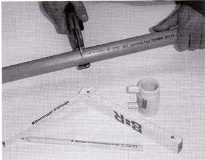
Fig. 1 Cut the pipe in a rectangular manner with plastic scissors or with a pipe cutter.
