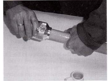
Fig. 3 On Bänninger Stabi-Pipes , the aluminium coating must be peeled off before jointing.
