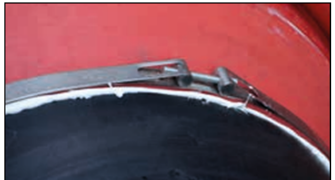
CaseCore Compenseal stainless steel straps used for pipe sizes up to OD 315 mm, Torque value 10 Nm
