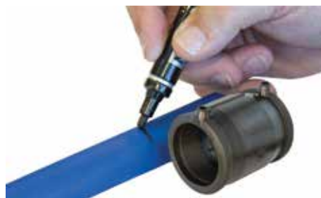
4. Witness mark correct insertion depth.
