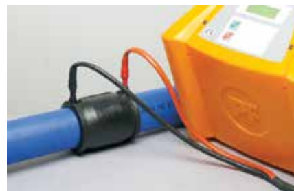
6. Connect welder leads onto fitting terminals (non specific). If using manual setting follow weld time as per label on fitting. Press start to commence weld cycle. Rising melt indicators confirm successful completion of weld. Remove leads and allow to cool without movement or strain on joint.
